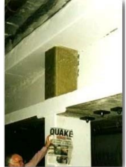
Figure 7. Retrofitted column at Hotel Nikko
